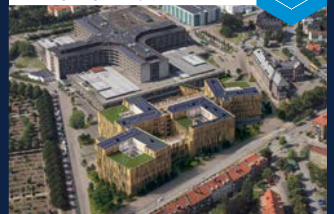
REGION: SCANDINAVIA Helsingborgs Hospital
